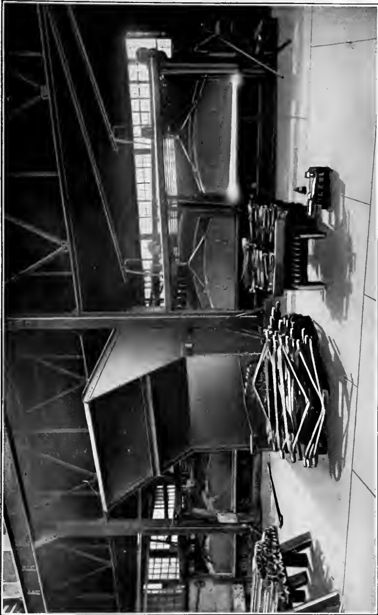
Plate-heating Furnace Arrangements.
